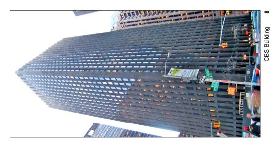
framing; instead, its structural system consists of a central core and a dense grid of columns around its exterior. The development site is north of this building across West 53rd Street.
