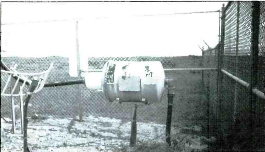
Fig. 7- Isocoupler used to couple FM antenna on top of TUK antenna to transmitter. It isolates tower from ground and FM transmitter, and prevents interreaction of FM signals and TUK's signals.
