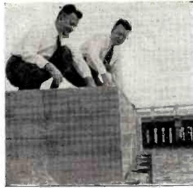
M. C. SCOTT (l), chief engineer, WIOD Miami, Fla., explains to J. Leonard Reinsch, managing director, Cox stations, details of the construction of a concrete anchor for one of the new hurricane-proof towers being built at WIOD's transmitter site in Biscayne Bay. Total weight of the concrete and steel in the three anchor foundations and the tower base foundation is 3,527,000 lbs.
