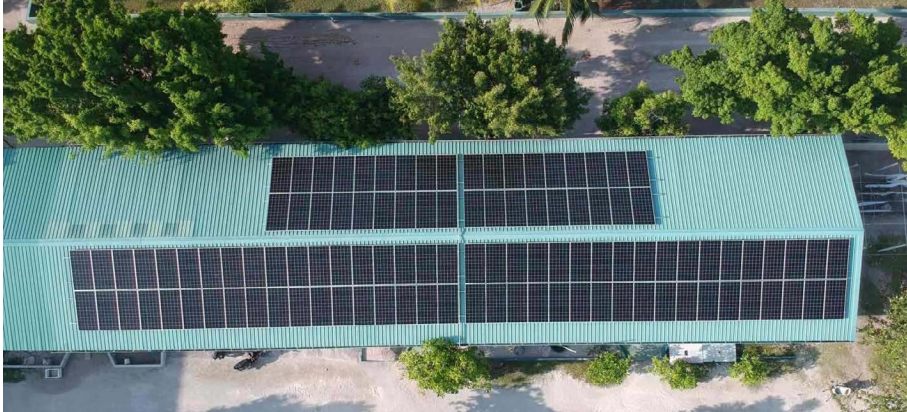
An aerial view of a solar-powered hospital in Maldives
