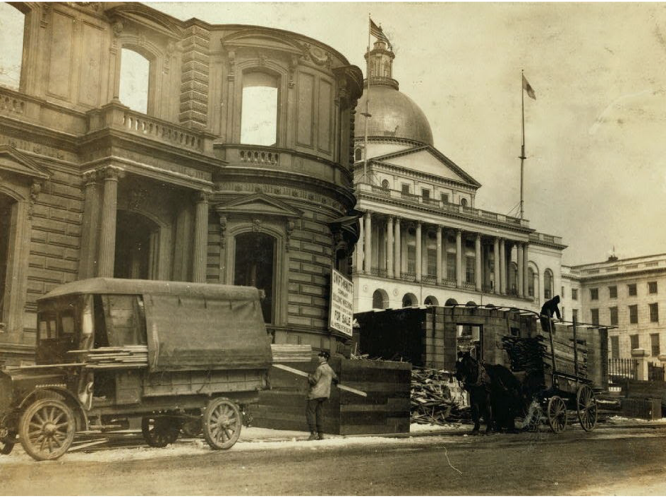
Taken 1917: Demolition of Townhouses to make room for the West Wing of the State House. We can see the Bulfinch front and the completed East Wing in this photo.
